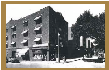
The Drake Court Annex with a glimpse of a neighboring park.
